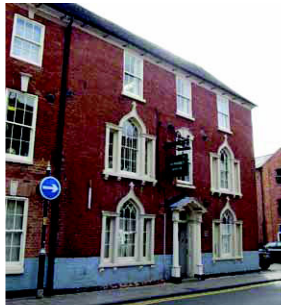
5 and 7 Worcester Road
