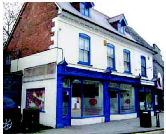
33, 35 and 37 Worcester Road
